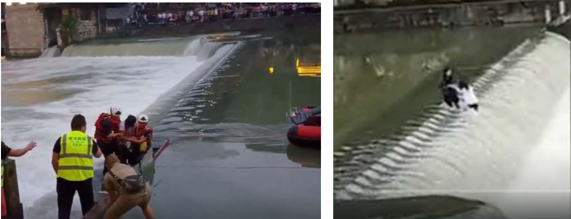
Wanrong River Dam, Jishou City (May 11, 2021)
