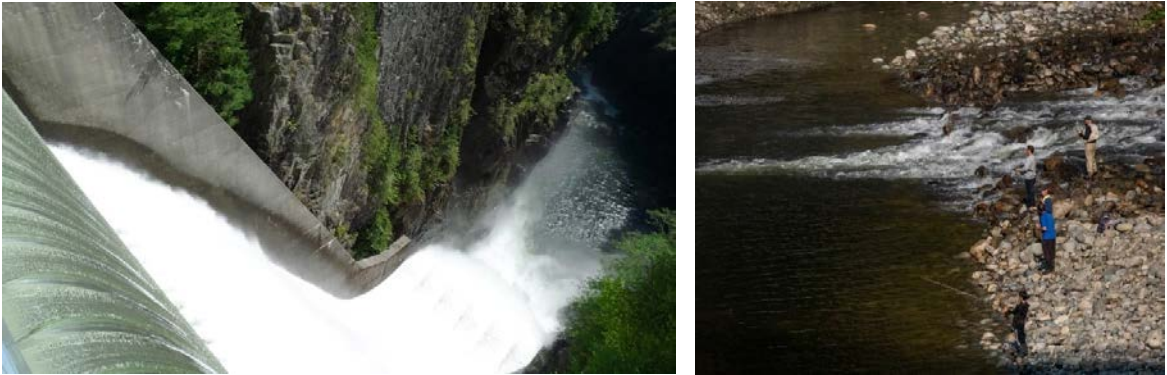
Cleveland Dam, Vancouver (October 1, 2020)
